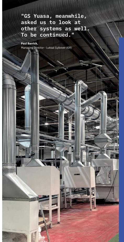
To meet the stringent emission standards, we chose 2 Keller PT 228 dust filters with the KLR Bran filter plate technology. Each of the 9 workstations on the production line has an airflow of 1 m/s from the operator to the dust filters.
