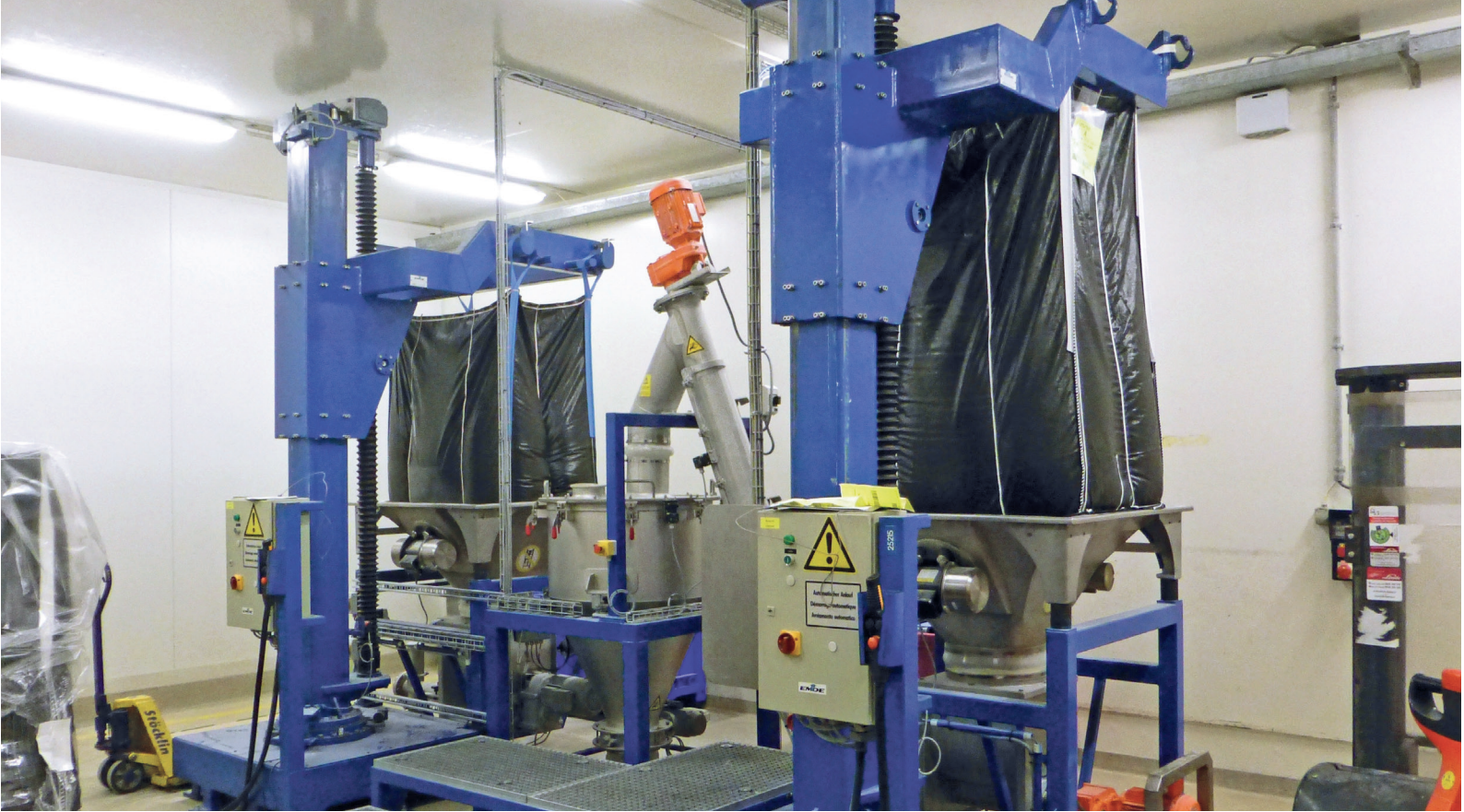
Big Bag emptying station type BE 1500 HSS with lift/swiveling column
