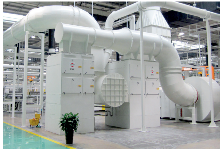
Dust extraction of a truck-engine production with a volume flow of 140 000 m³/h
